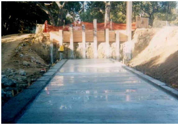
Launch slab - looking towards backstop
