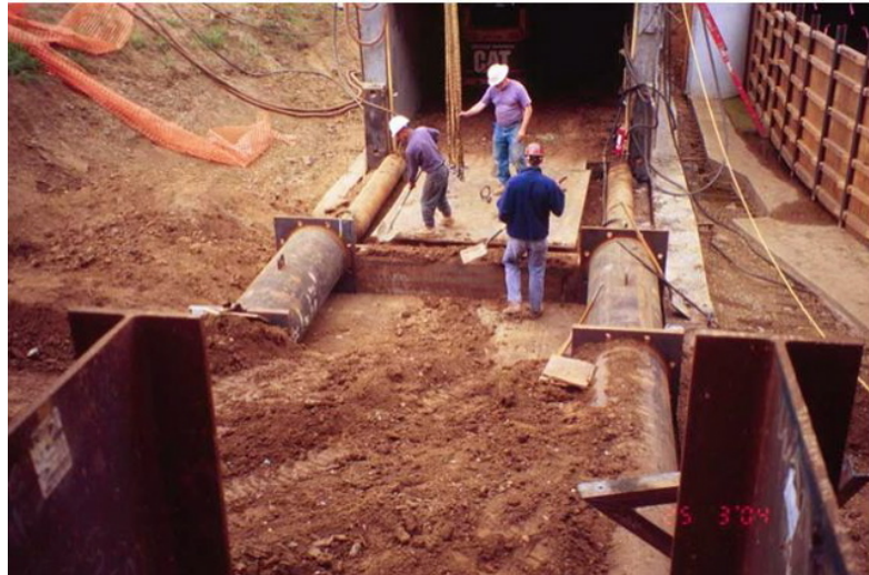
Adding thrust columns after jacking 8'
