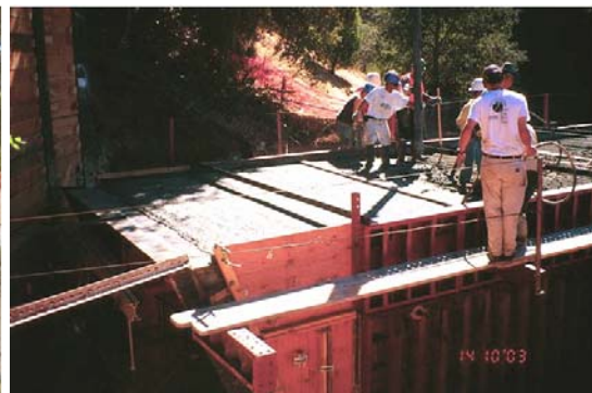
Casting roof & walls of box
