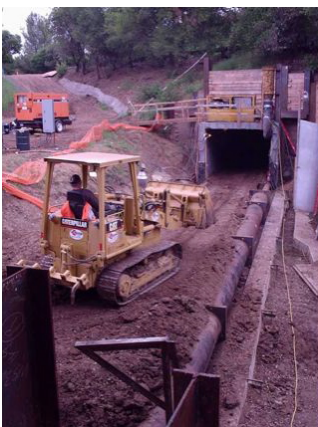
Mucking tunnel w/Cat 933
