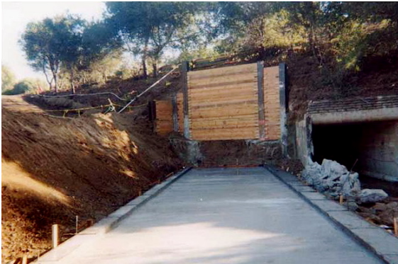
Launch slab looking at portal wall
