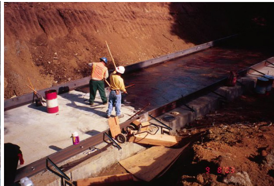
Applying grease to launch slab
