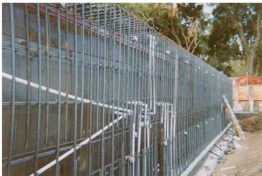
Slurry piping & rebar in box walls
